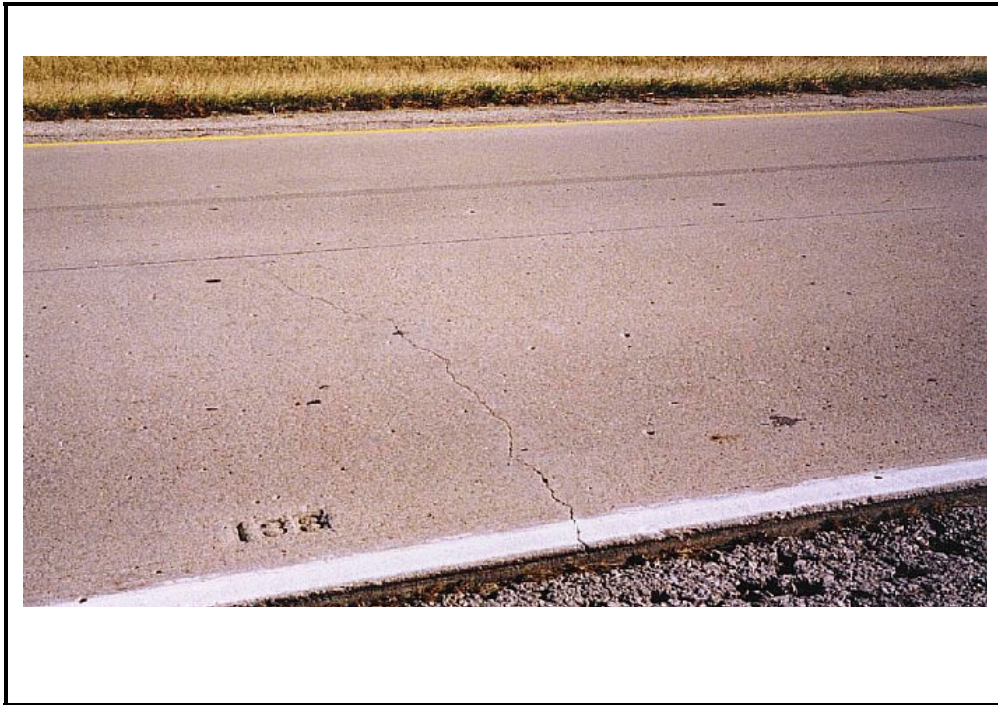
Photo C-16. Transverse Cracking in Jointed Concrete Pavement, Low Severity
