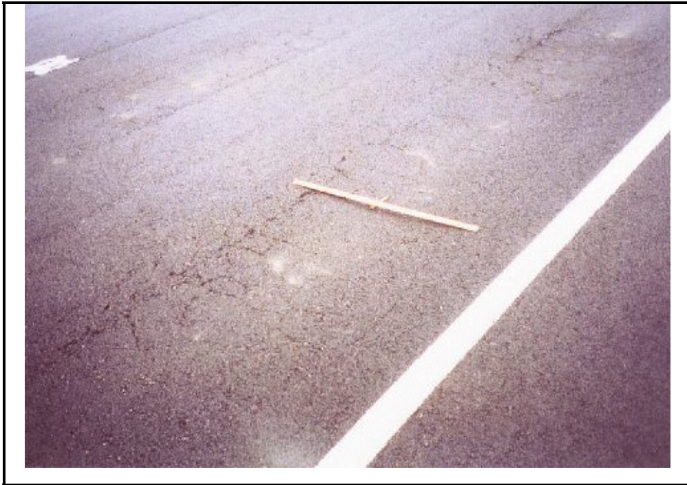
Photo A-10. Rutting in Flexible Pavement, Medium Severity
