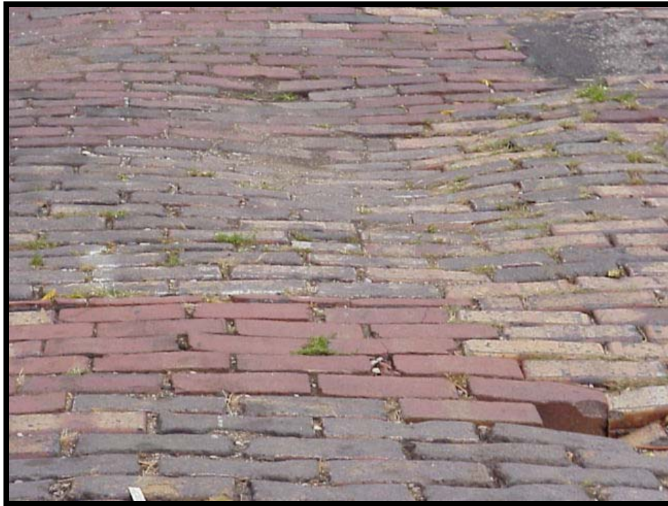
Photo F-15. Settlement in Brick Pavers, High Severity
