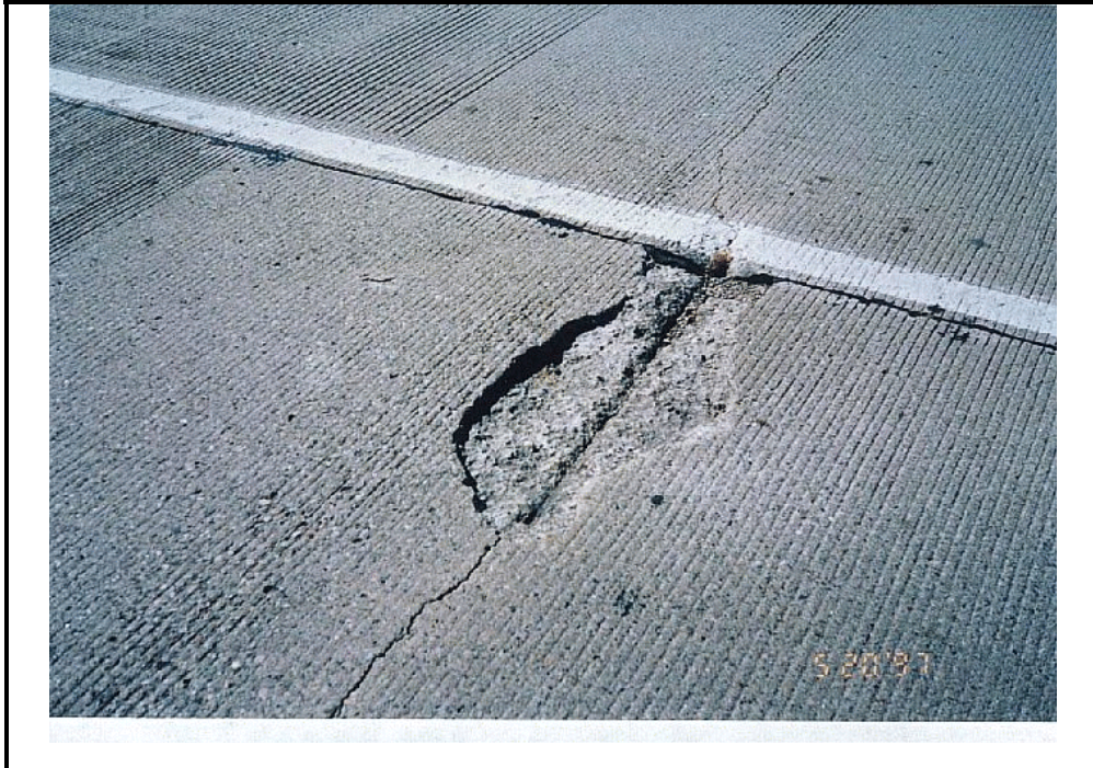
Photo C-15. Pressure Damage in Jointed Concrete Pavement
