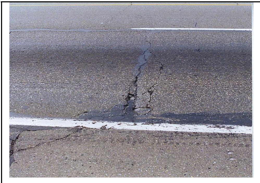
Photo E-25 . Crack sealing Deficiency in Local Pavement, Cracks not sealed sufficiently
