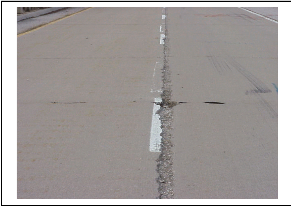
Photo C-3. Longitudinal Joint Spalling in Concrete Pavement, High Severity
