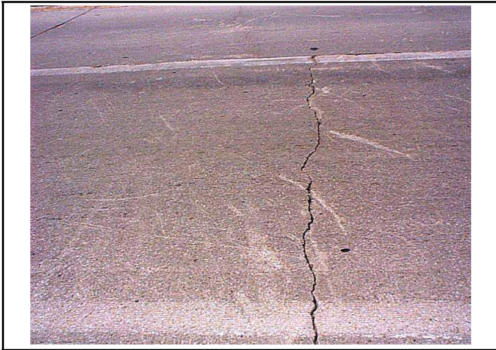
Photo C-13. Transverse Cracking - Plain Concrete in Jointed Concrete Pavement, Medium Severity
