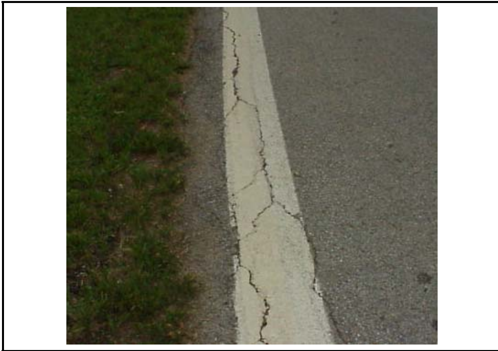
Photo E-21 . Edge Cracking in Local Pavement, Medium Severity
