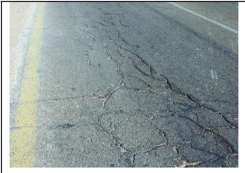
Photo A-16. Wheel Track Cracking in Flexible Pavement, High Severity
