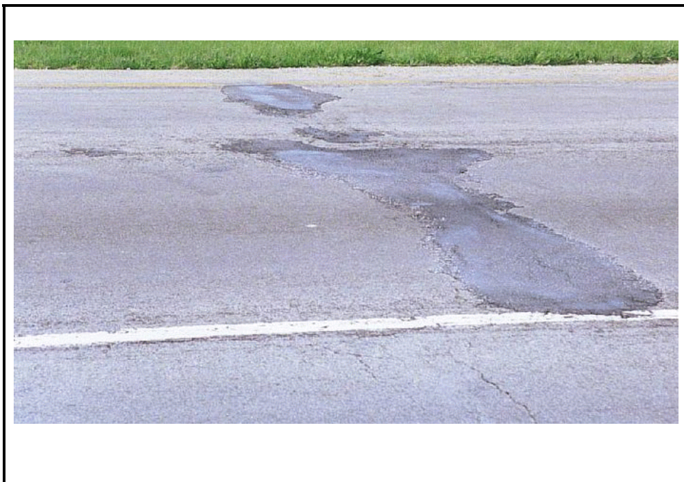
Photo A-6. Patching in Flexible Pavement, High Severity
