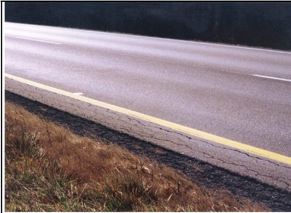
Photo A-21. Edge Cracking in Flexible Pavement, Medium Severity
