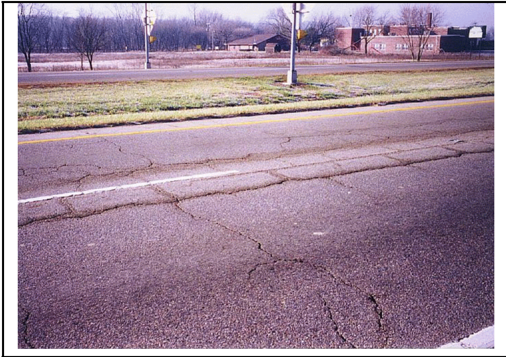
Photo B-21. Crack Sealing Deficiency in Composite Pavement, Unsealed Cracks
