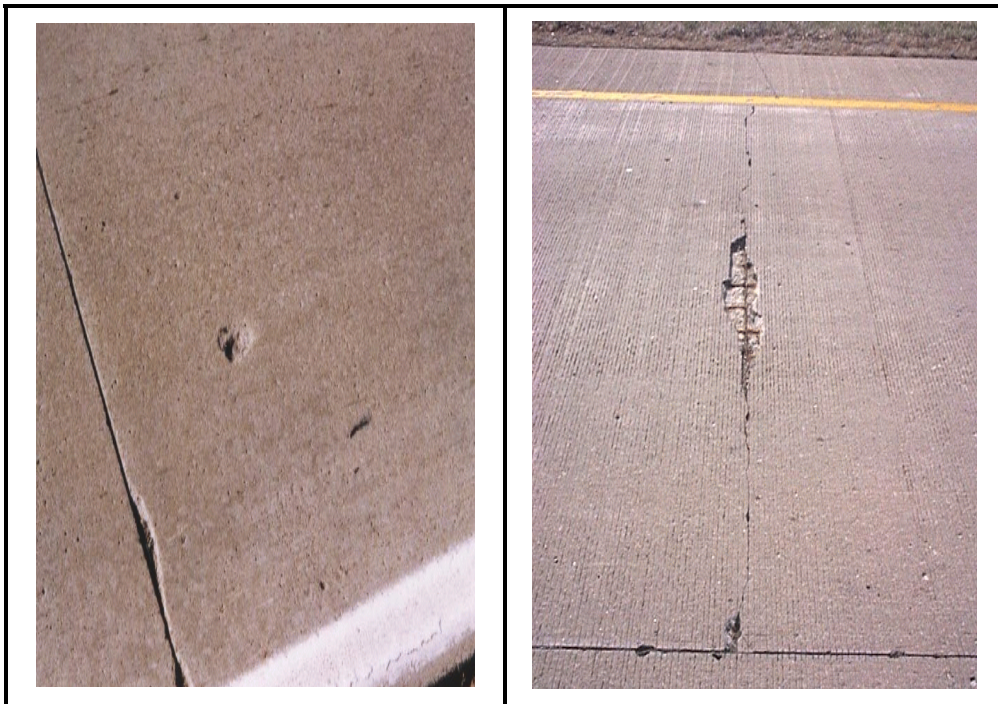
Photo C-2. Surface Deterioration in Jointed Concrete Pavement, Popouts and High Steel
