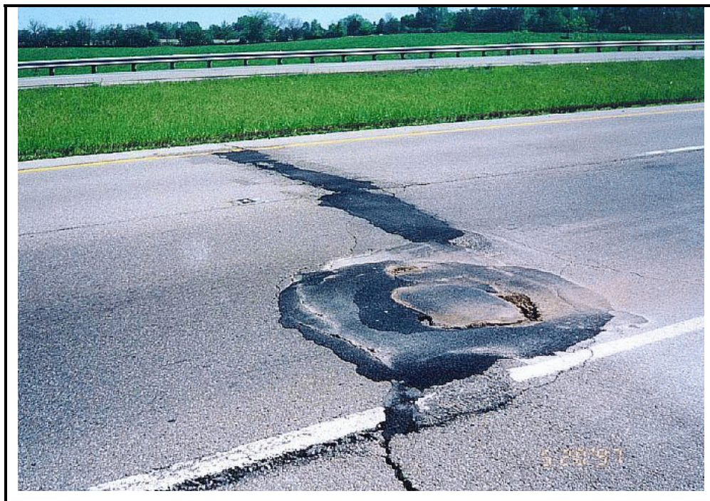
Photo B-12. Pumping in Composite Pavement
