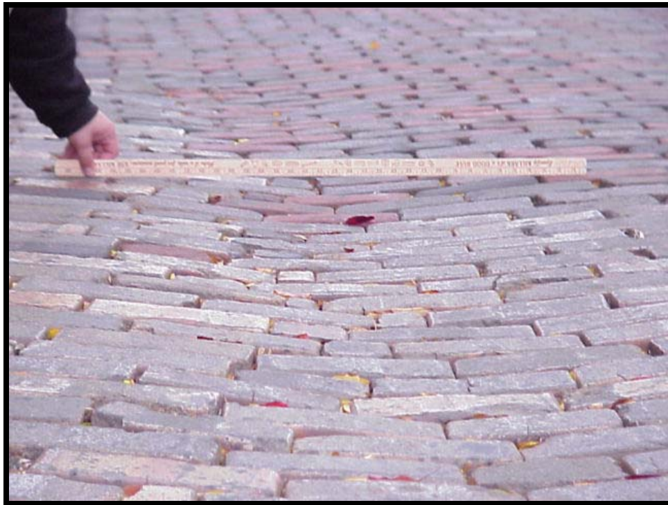
Photo F-9. Rutting in Brick Pavers, Medium Severity
