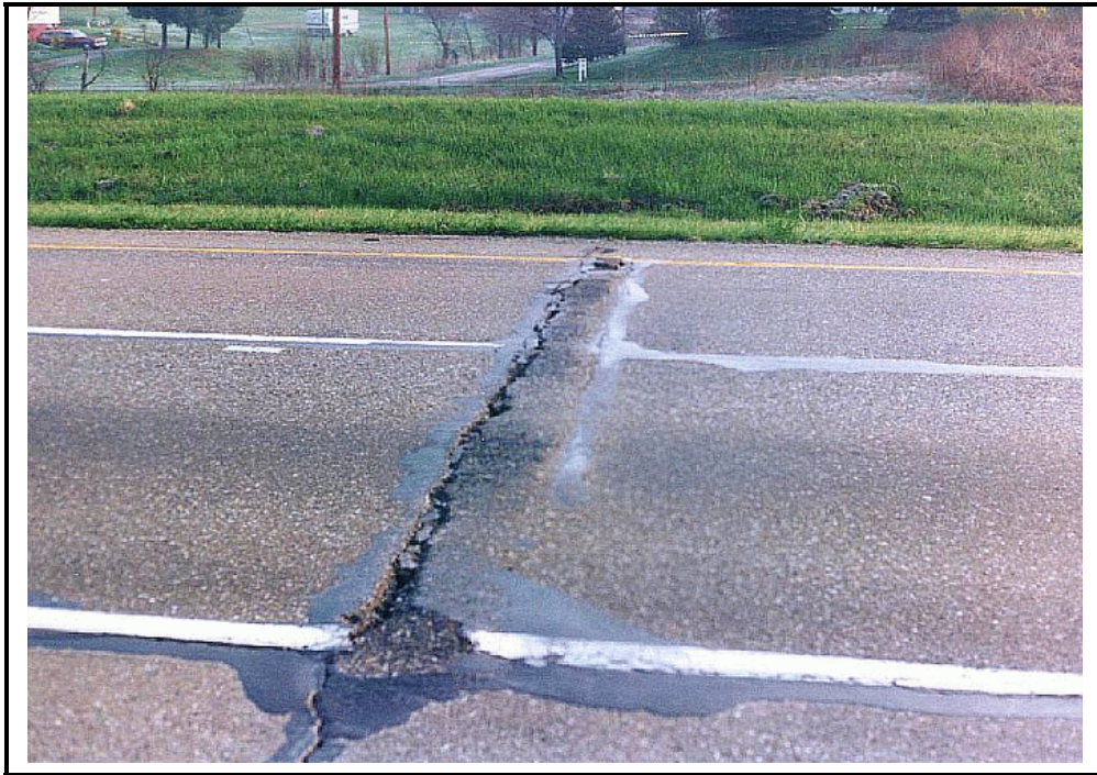
Photo E-23 . Pressure Damage/Upheaval in Local Pavement, Medium Severity
