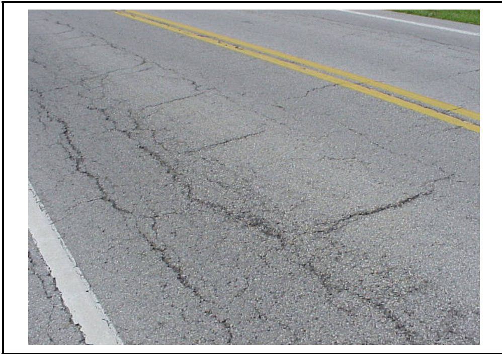
Photo A-17. Block and Transverse Cracking in Flexible Pavement, Medium Severity
