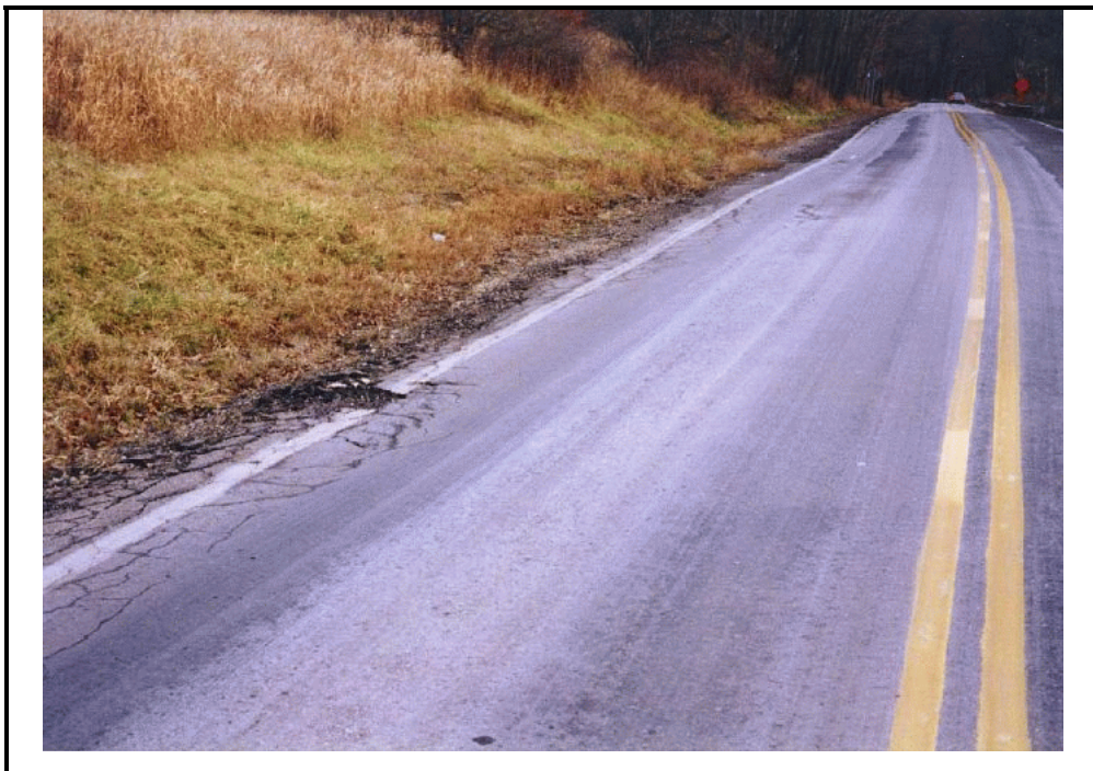
Photo E-22 . Edge Cracking in Local Pavement, High Severity
