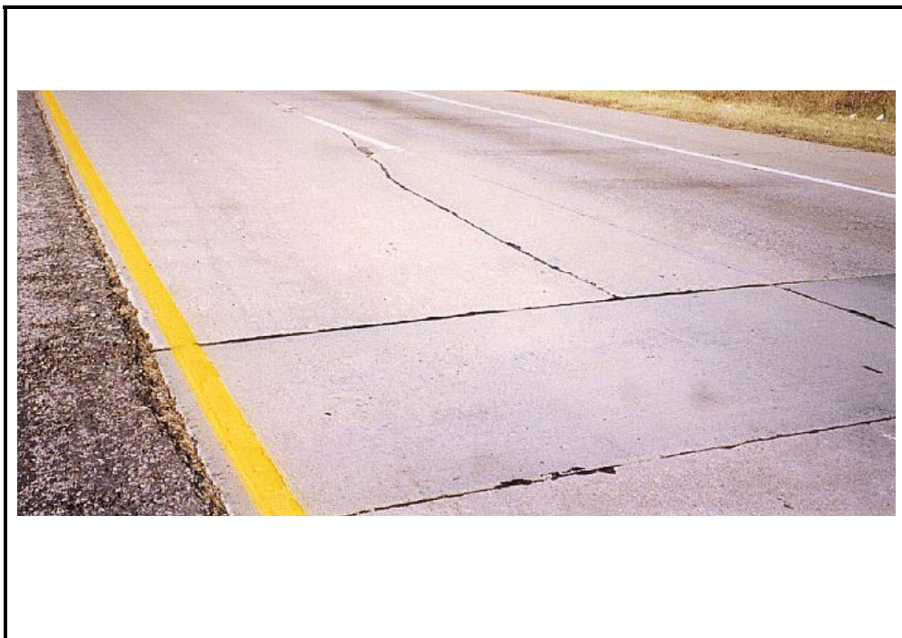
Photo C-19. Longitudinal Cracking in Jointed Concrete Pavement, Medium Severity
