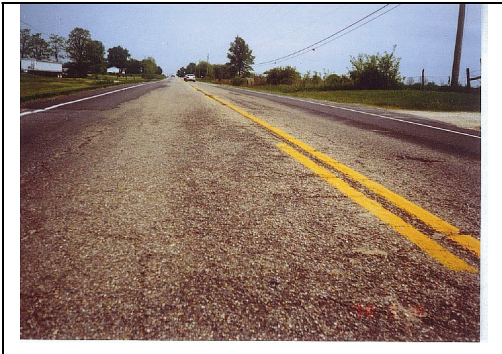
Photo B-2. Raveling in Composite Pavement, High Severity
