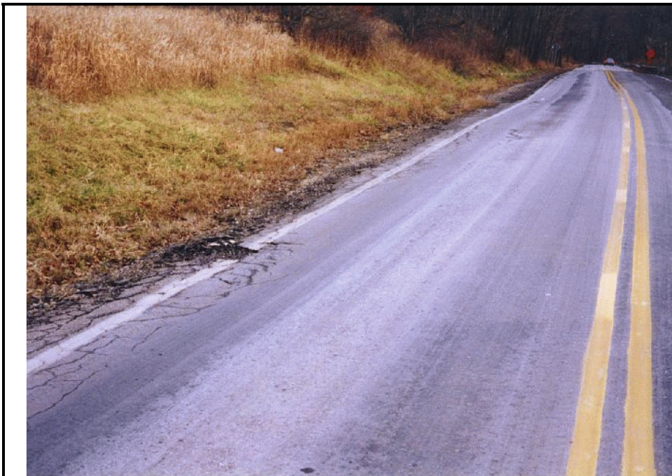
Photo A-21. Edge Cracking in Flexible Pavement, Medium Severity
