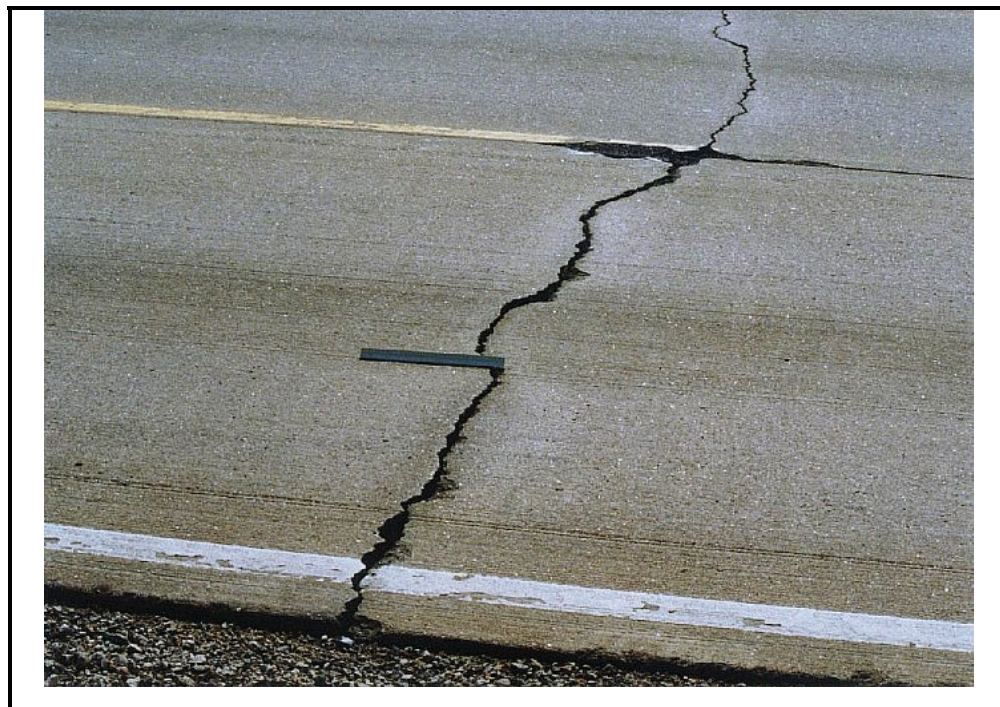
Photo C-9. Faulting in Jointed Concrete Pavement
