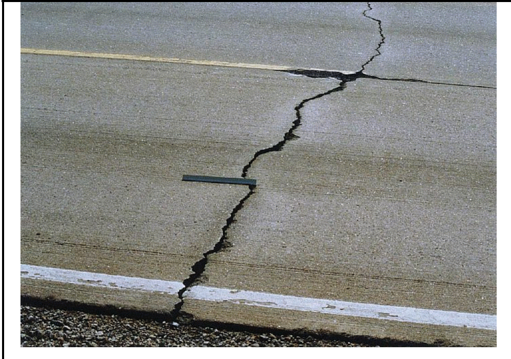
Photo C-17. Transverse Cracking in Jointed Concrete Pavement, High Severity
