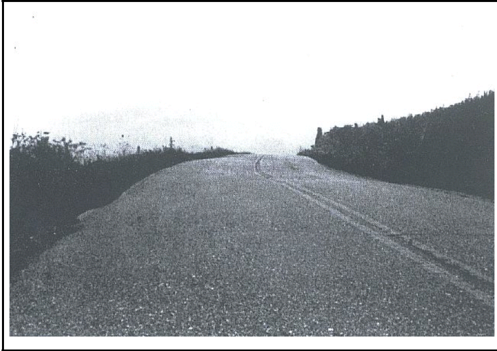
Photo A-12. Settlement in Flexible Pavement, Low Severity
