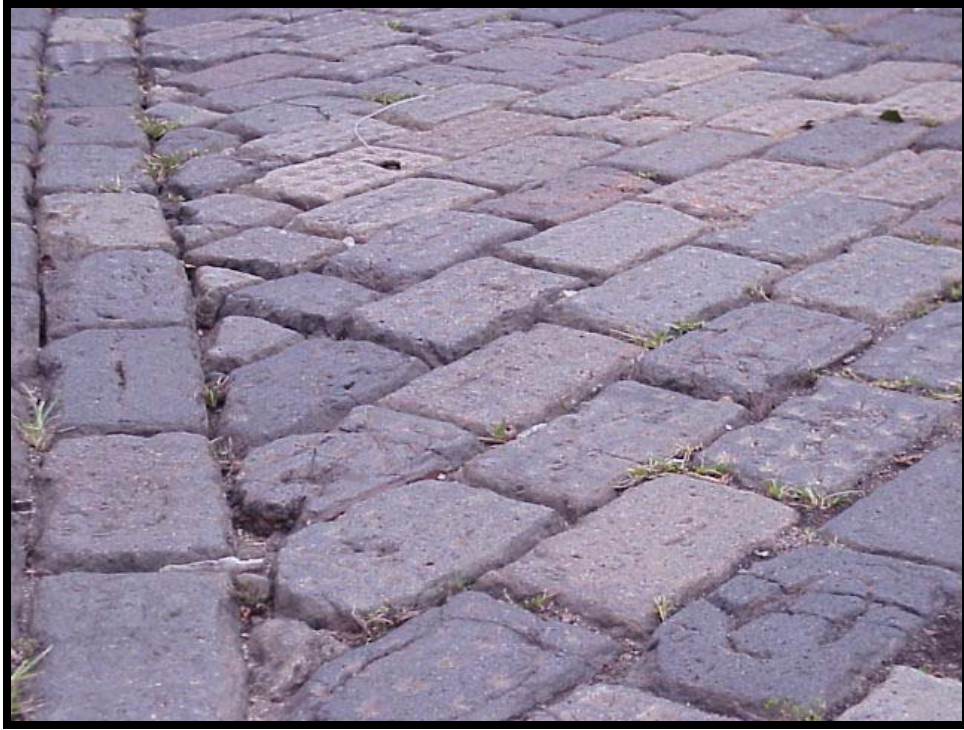
Photo F-13. Joint Erosion in Brick Pavers, Medium Severity
