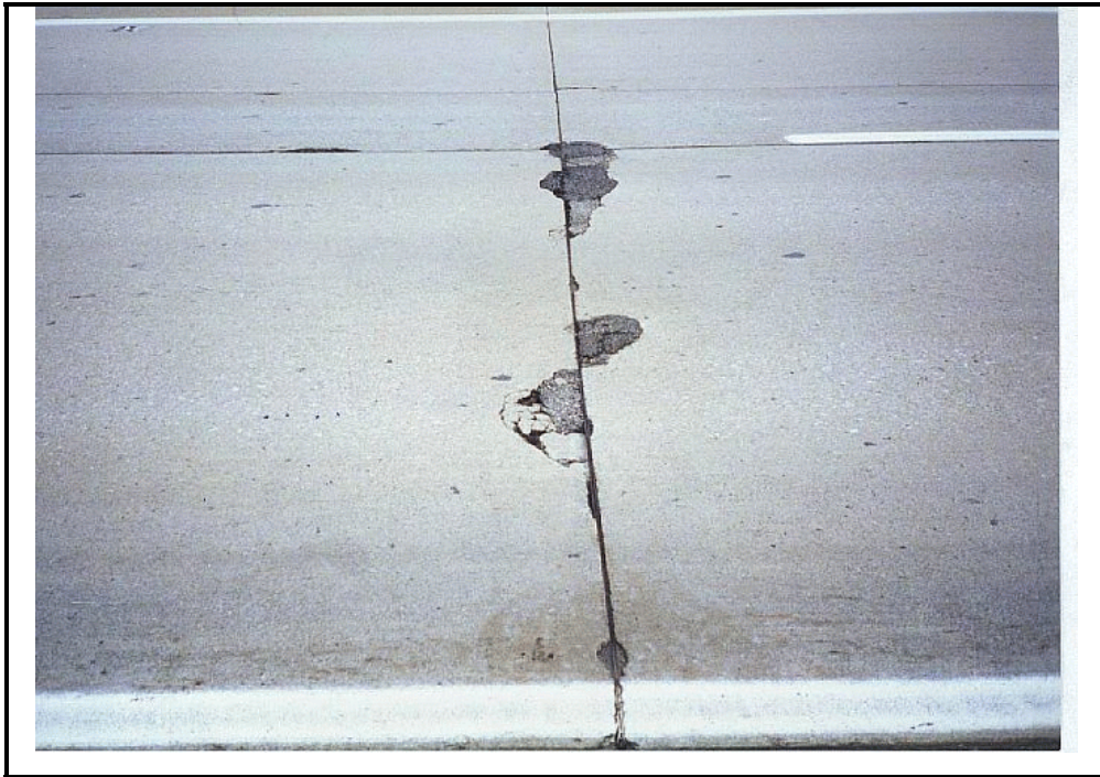
Photo C-4. Patching in Jointed Concrete Pavement, Low Severity
