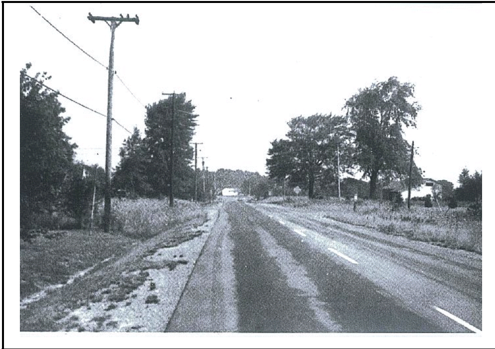
Photo A-3. Bleeding in Flexible Pavement, High Severity
