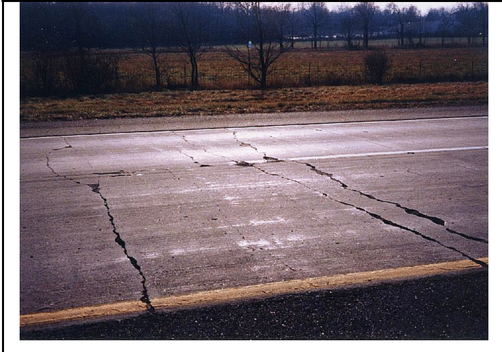
Photo D-11. Transverse Cracks in CRC Pavement, Medium Severity
