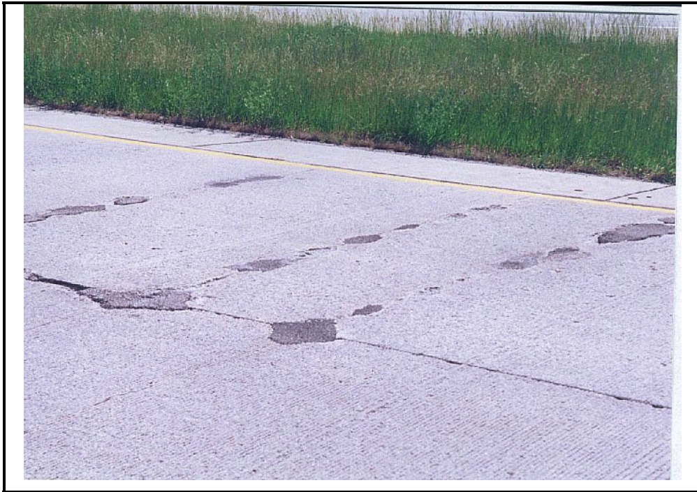
Photo D-5. Patching in CRC Pavement, Low Severity
