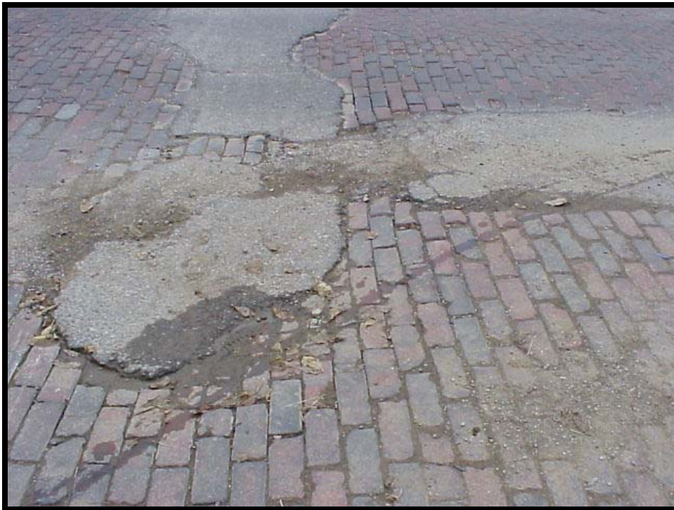
Photo F-8. Pumping in Brick Pavers
