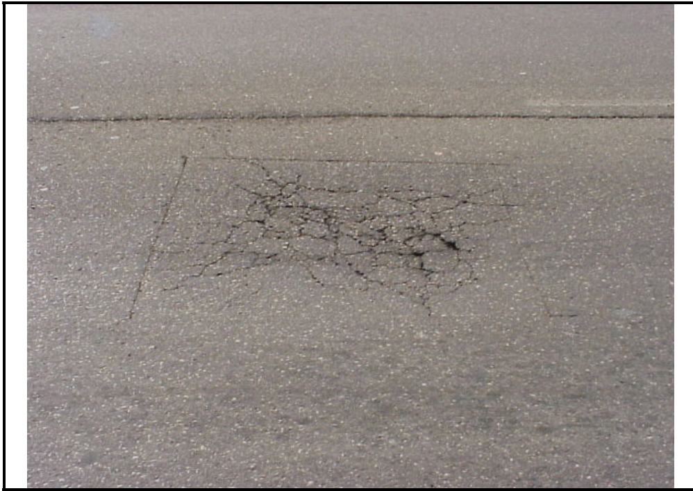
Photo B-24. Punchouts in Composite Pavement, Low Severity
