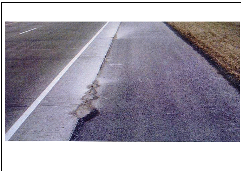
Photo C-7. Pumping in Jointed Concrete Pavement, Low Severity
