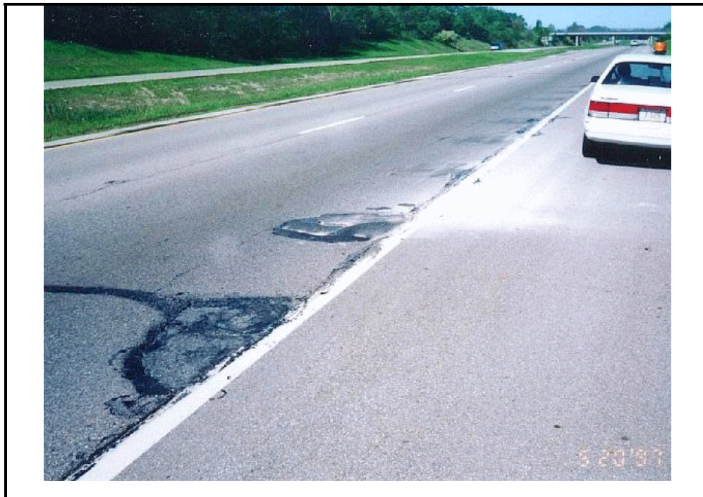
Photo B-11. Pumping in Composite Pavement
