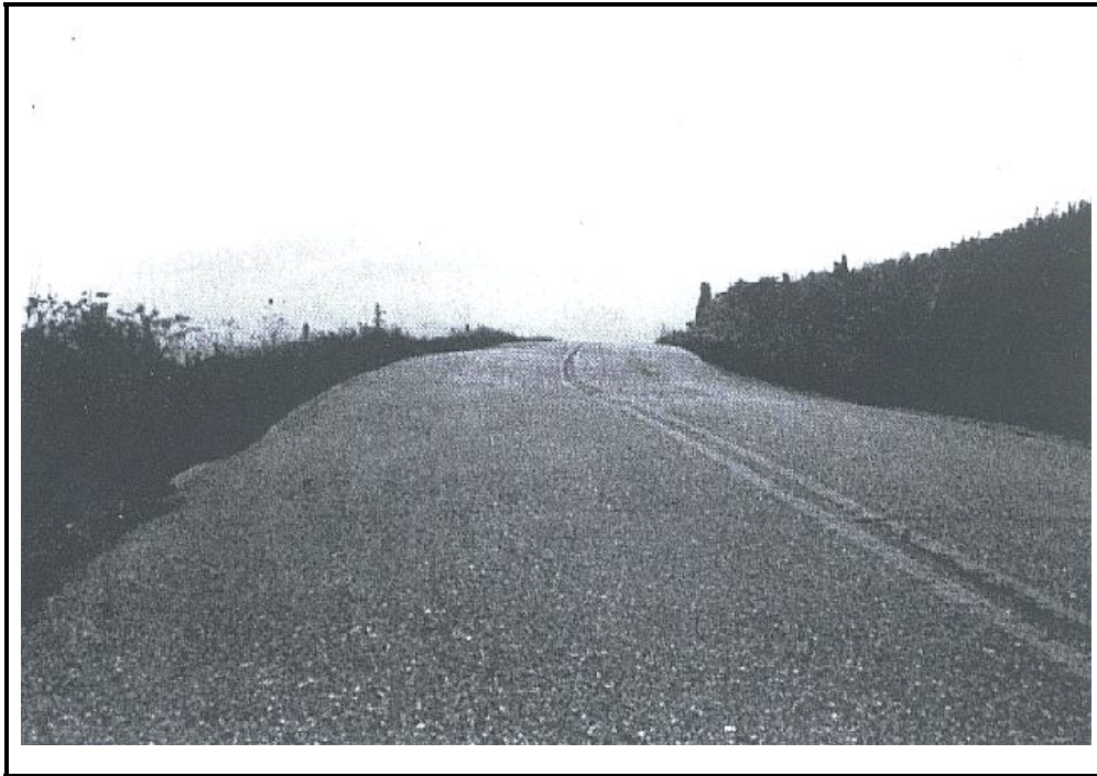
Photo E-14 . Settlement in Local Pavement, Low Severity
