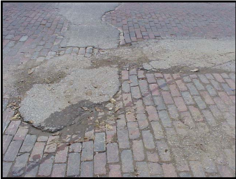
Photo F-5. Patching in Brick Pavers, High Severity
