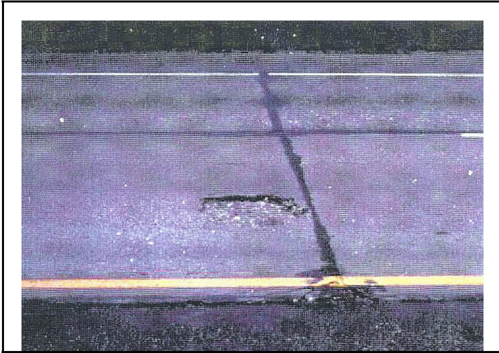
Photo D-18. An Example of Pressure Damage in Jointed Concrete Pavement . Pressure Damage in CRCP is similar to as shown above.
