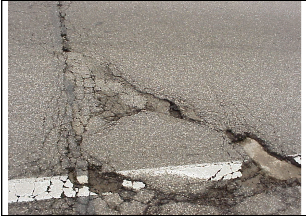
Photo B-23. Corner Break in Composite Pavement, High Severity
