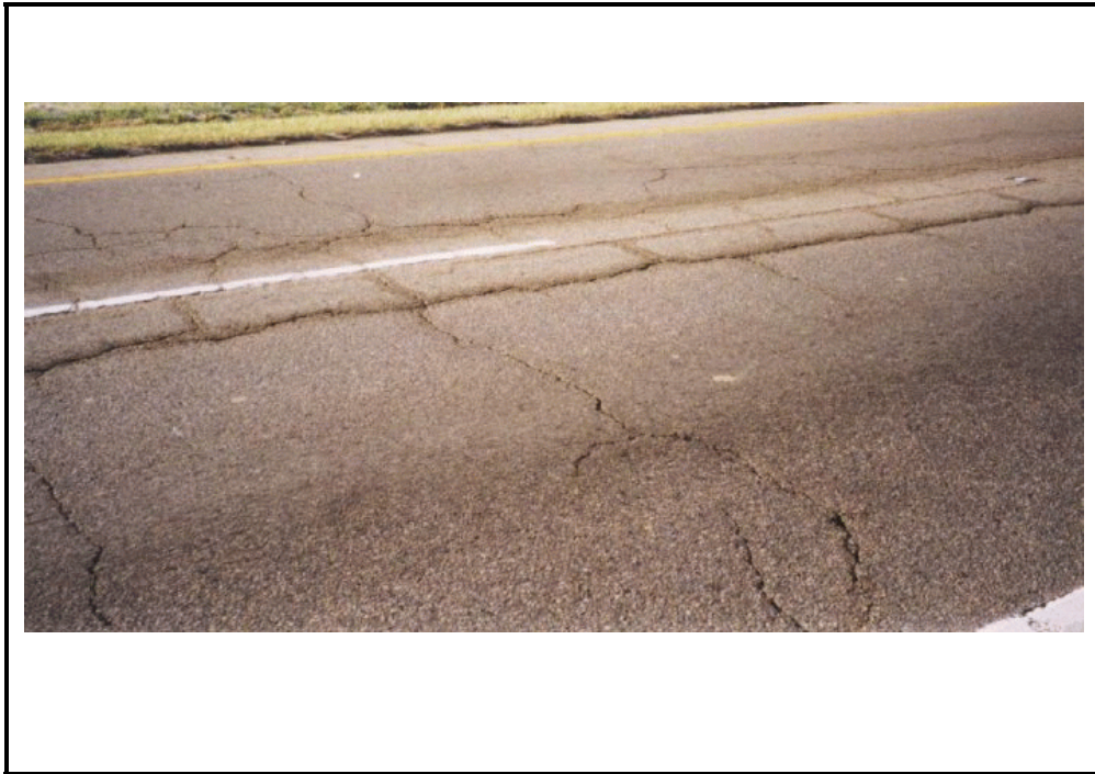
Photo E-24 . Crack Sealing Deficiency in Local Pavement, Unsealed Cracks
