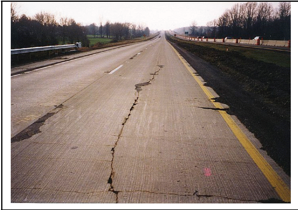
Photo D-12. Longitudinal Cracking in CRC Pavement, Medium Severity
