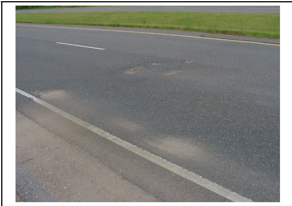
Photo B-25. Punchouts in Composite Pavement, Medium Severity Error!Bookmark not defined.
