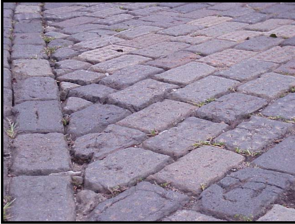
Photo F-11. Corrugations in Brick Pavers, High Severity
