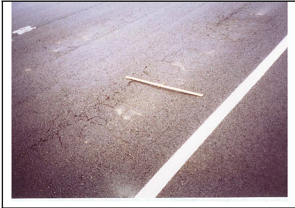
Photo B-9. Rutting in Composite Pavement, Medium Severity
