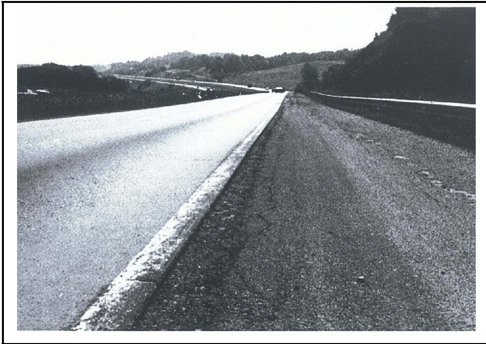
Photo D-9. Settlement in CRC Pavement
