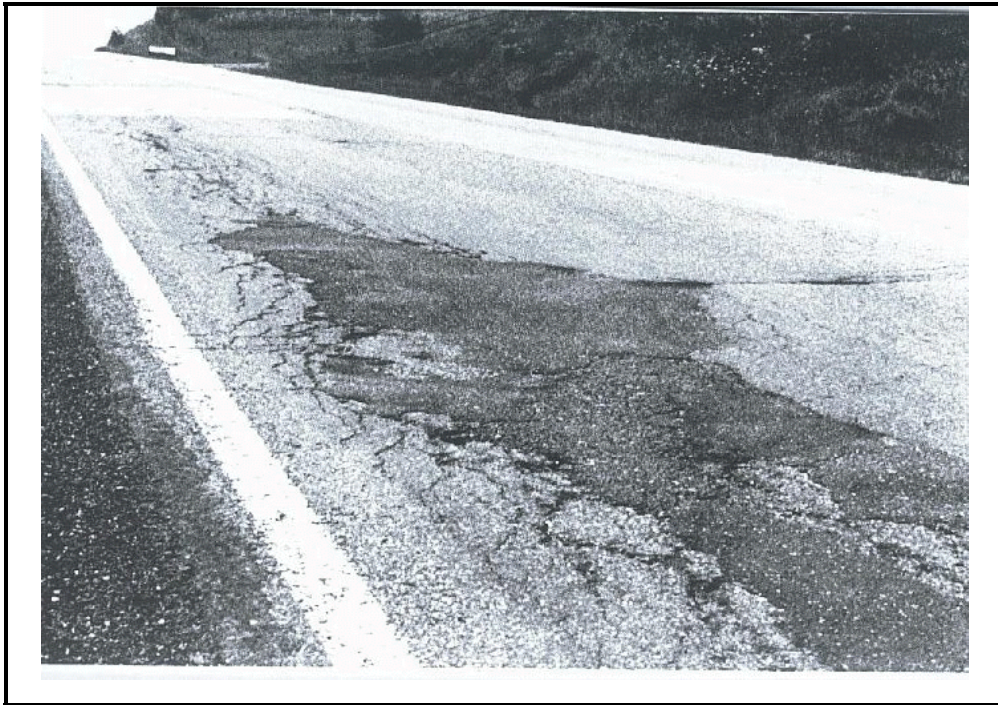
Photo E-5 . Patching in Local Pavement, High Severity
