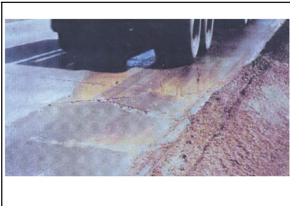
Photo C-6. Pumping in Jointed Concrete Pavement, High Severity
