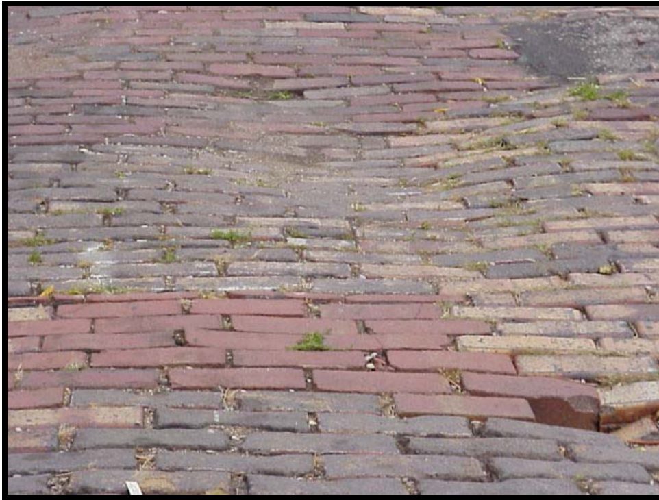
Photo F-7. Pumping in Brick Pavers
