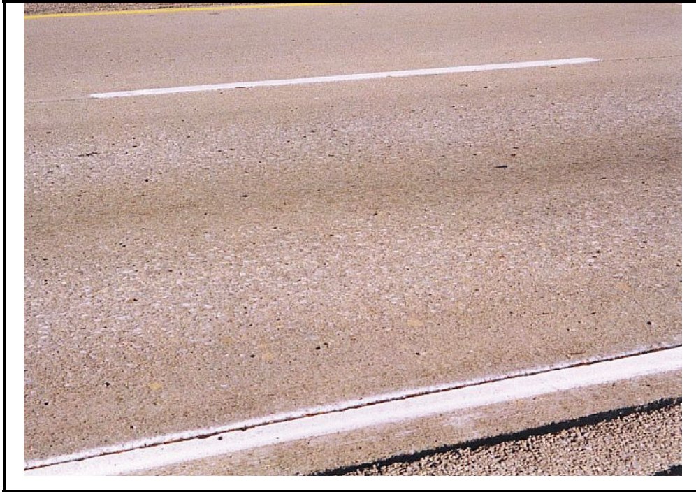
Photo D-1. Surface Deterioration in CRC Pavement, Medium Severity
