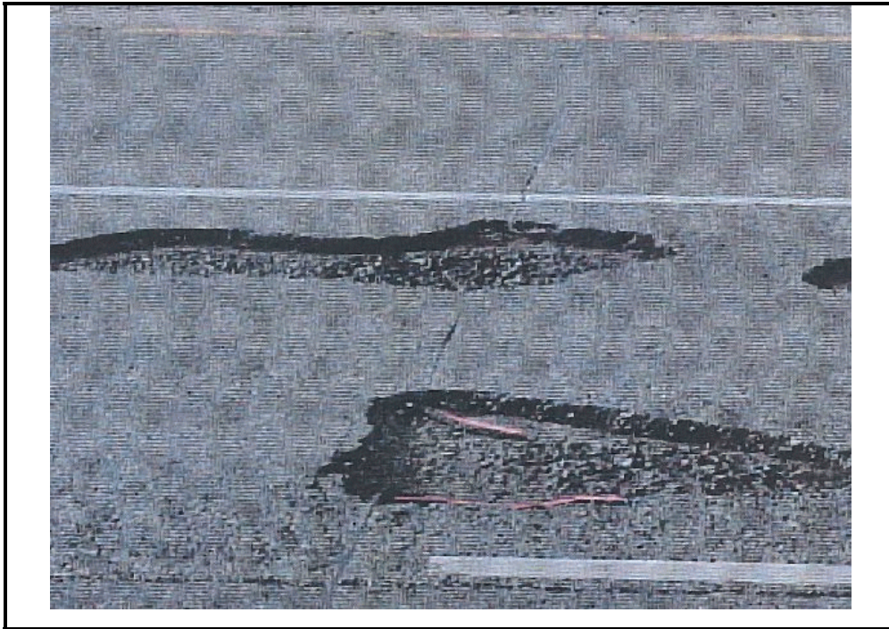
Photo B-7. Surface Disintegration in Composite Pavement
