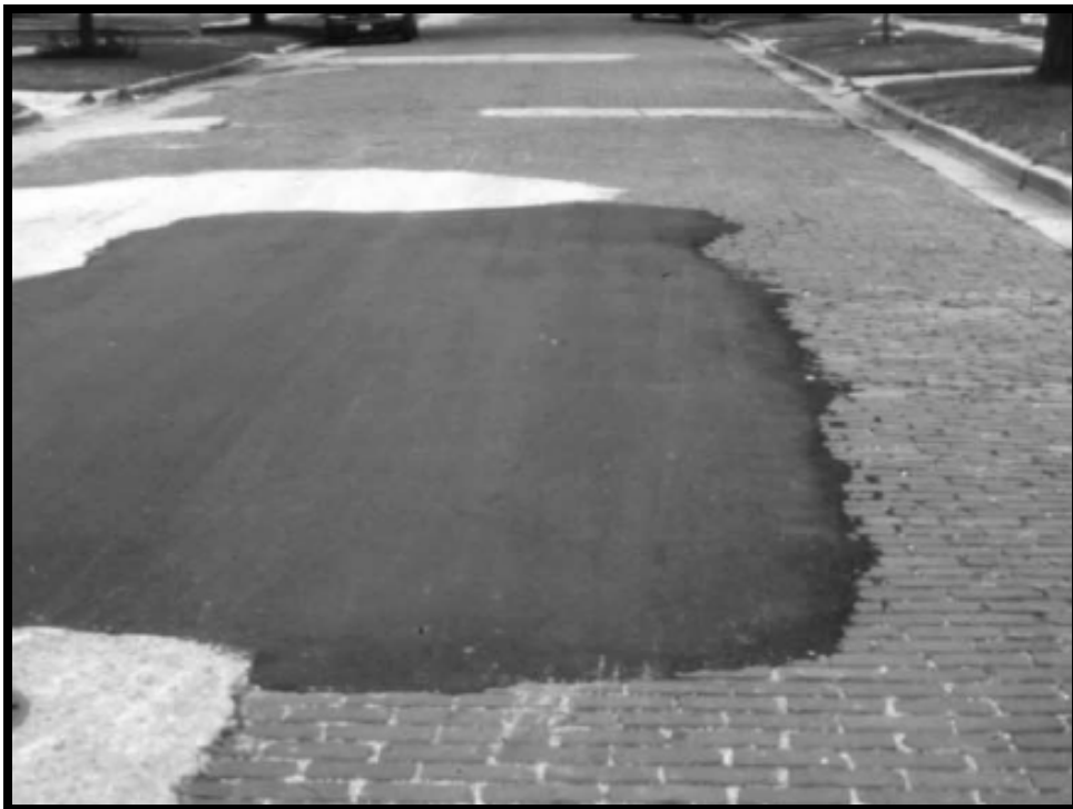
Photo F-6. Patching in Brick Pavers, High Severity
