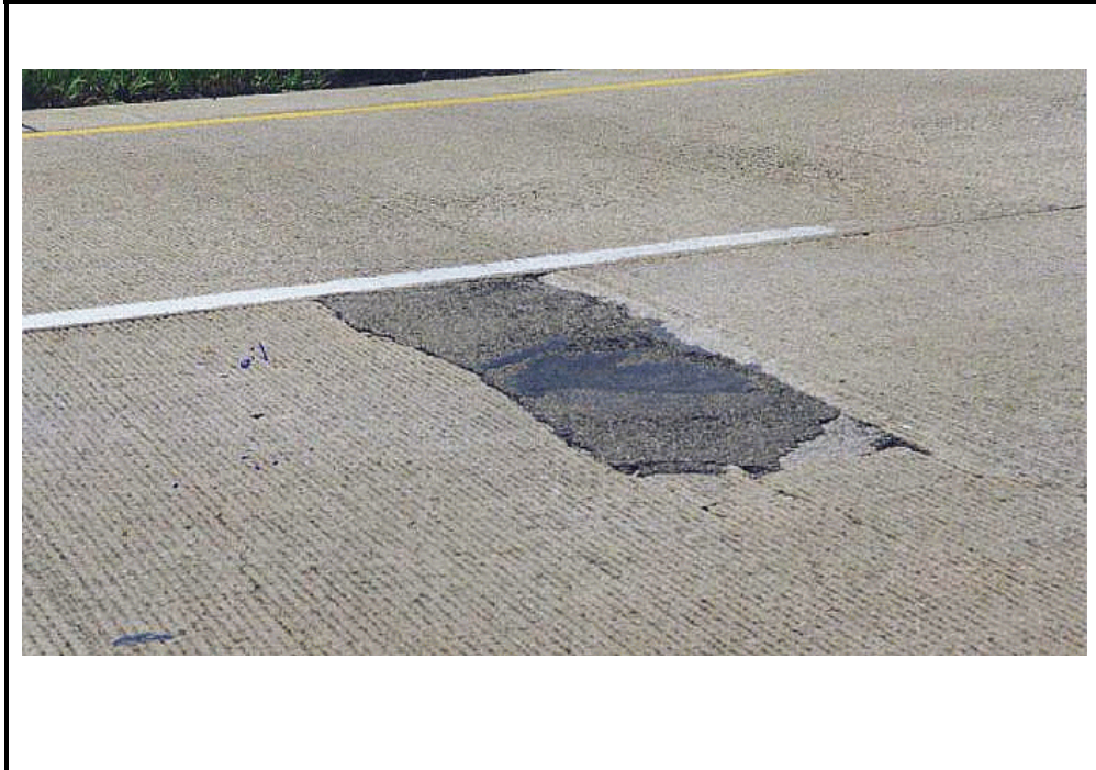
Photo C-5. Patching in Jointed Concrete Pavement, High Severity
