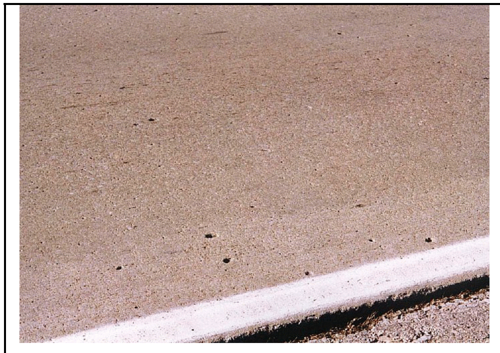
Photo D-4. Popouts in CRC Pavement
