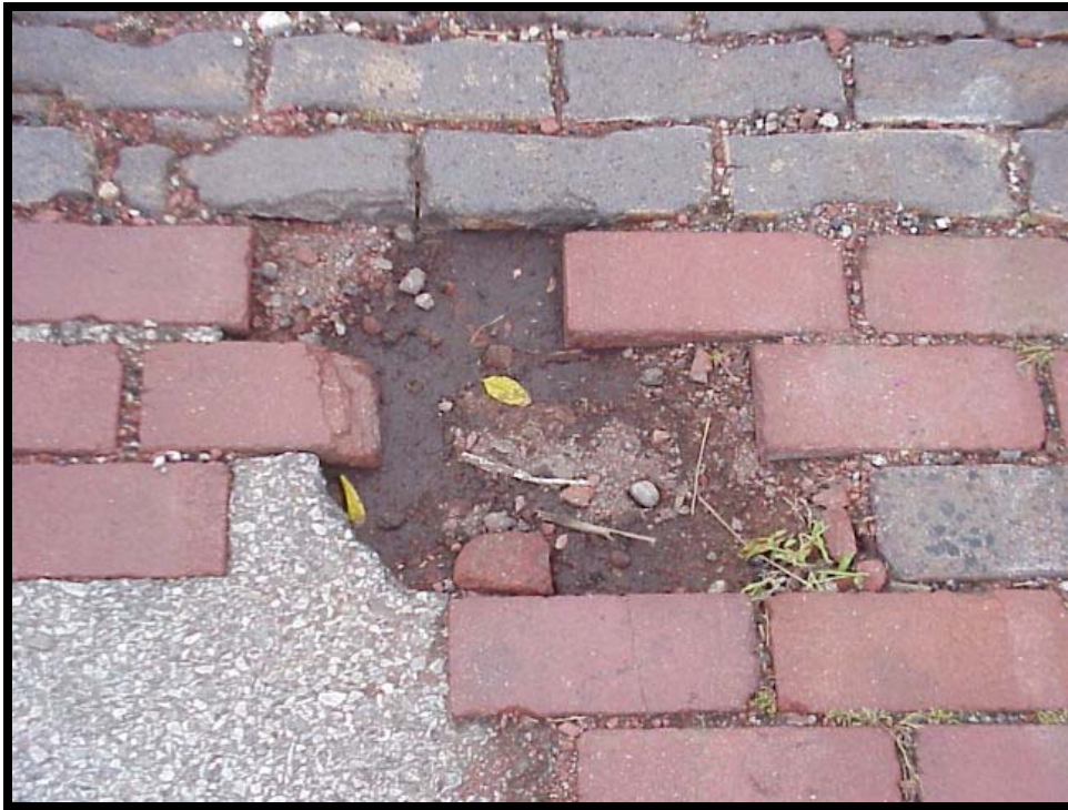
Photo F-1. Brick Deterioration in Brick Pavers, Medium Severity
