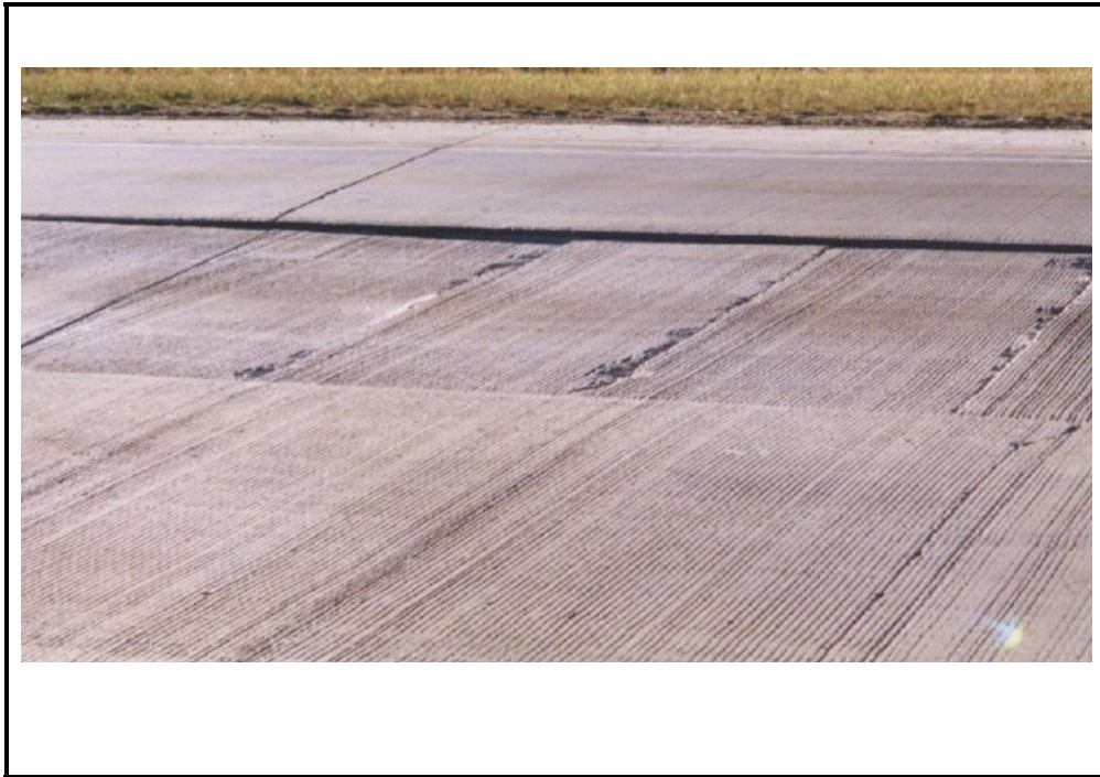
Photo C-10. Settlements in Jointed Concrete Pavement, Medium Severity
