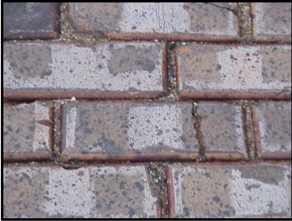
Photo F-3. Discoloration on Brick Pavers
