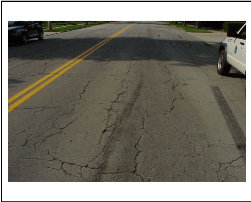
Photo E-11 . Map Cracking in Local Pavement, Medium Severity
