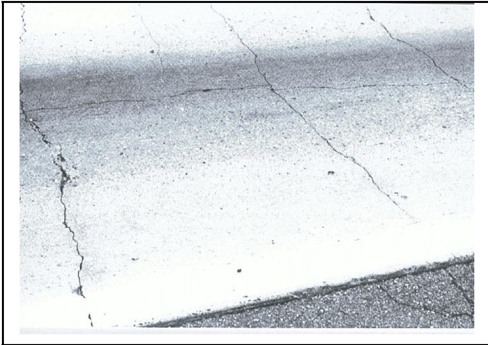
Photo D-14. Punchouts in CRC Pavement, Medium Severity
