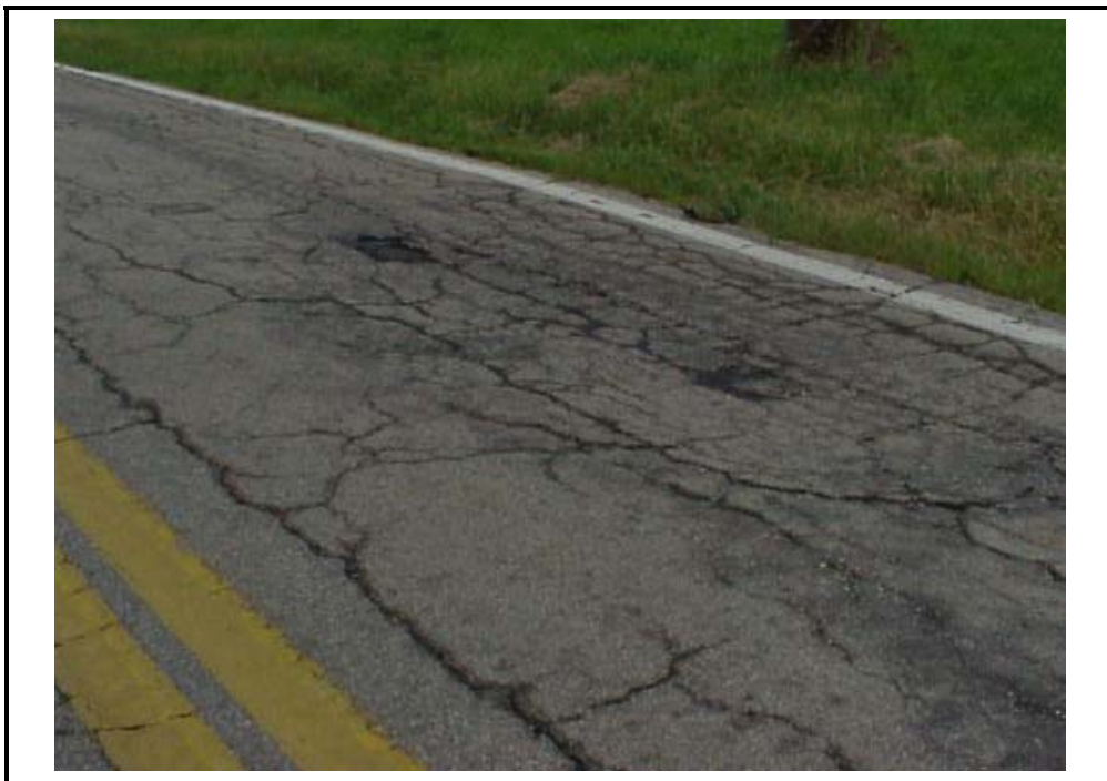
Photo E-19 . Wheel Track Cracking in Local Pavement, High Severity
