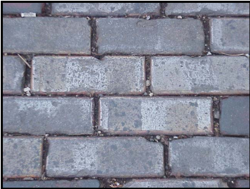
Photo F-4. Discoloration on Brick Pavers
