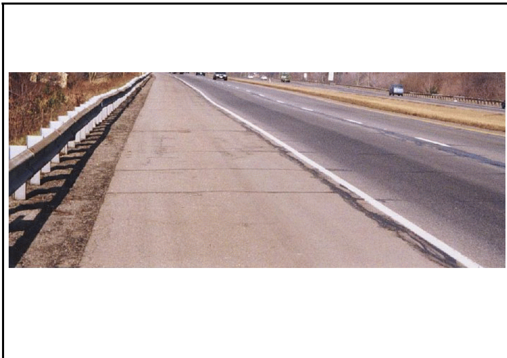
Photo E-15 . Settlement in Local Pavement, Medium Severity
