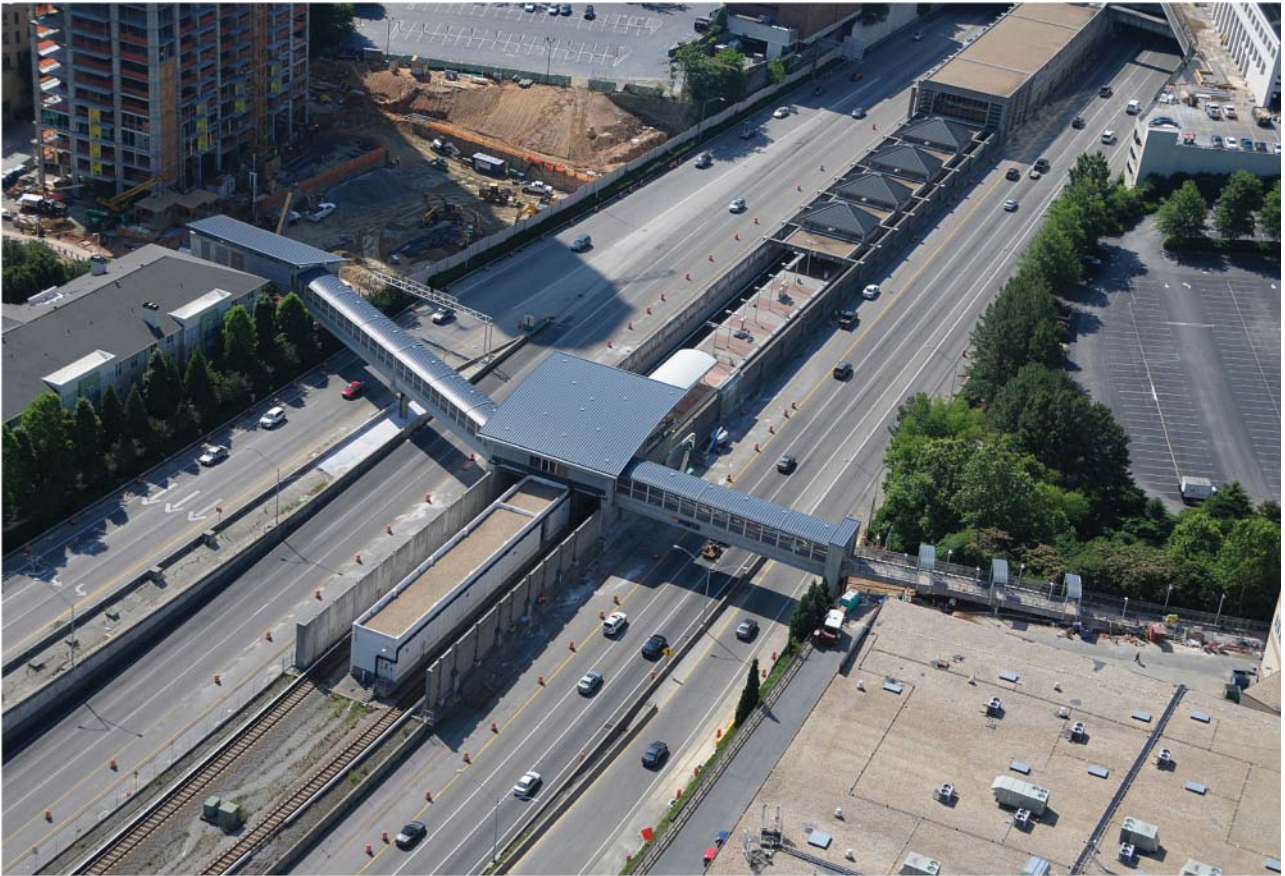
Figure 12-32. Pedestrian Access to Center Freeway Rapid Transit Station, Atlanta
