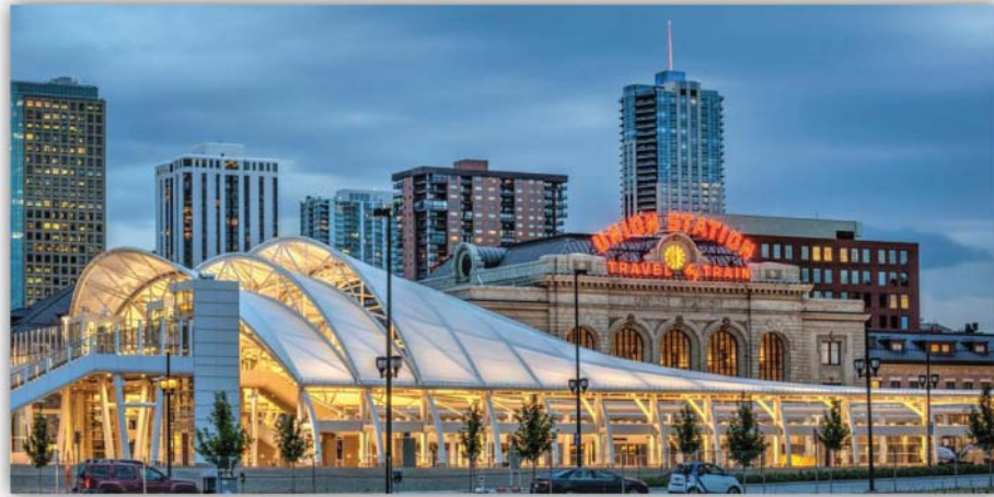
Figure 12-33. Denver's Union Station
