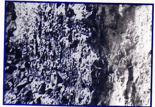
Figure 8 Sidewall Biomat in an Actual Trench
