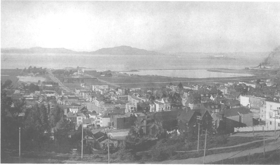
FIG. 9. Photograph of the Marina area taken in April (?) 1912. Shortly after the photograph was taken the cove in the right middle ground was hydraulically filled for the Panama-Pacific International Exposition. Sand was pumped from the bottom of the Bay, transported by pipeline, and discharged into the cove. The pond in the left part of the photo is now part of the lagoon at the Palace of Fine Arts. Next to the pond is Baker Street, and then Broderick Street. Photo courtesy of Archives, San Francisco Main Library.
